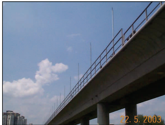
ALS-100 air terminals Singapore Rail Line
